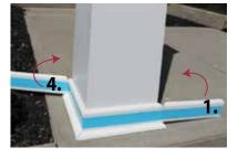
5 Unfold panel #1 and #4 into final position.
