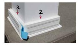
4 Slide #3 skirt against column. Bring #2 into contact with column. Press firmly.
