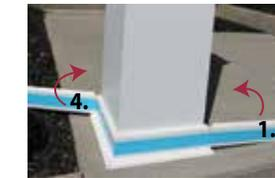
**5** Unfold panel #1 and #4 into final position. **NOTE:** Extra blue support tape can be used to hold the last corner together.
