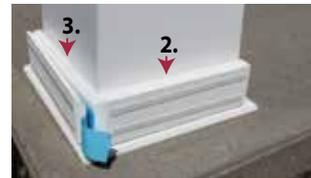
**4** Slide #3 skirt against column. Bring #2 into contact with column. Press firmly.
