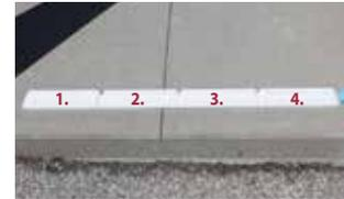
1 Take adhesive backing off panel #1, #2 and #4 (keep backing on #3 panel to allow for positioning).
